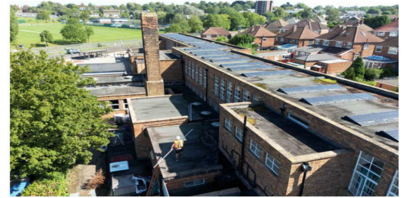
Remedial work being carried out at Mayflower primary school in Leicester, which has been affected by Raac. Photograph: Jacob King/PA
